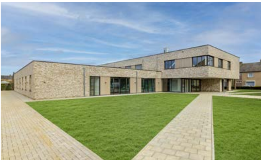
► Medical office building - Sittard (NL)
