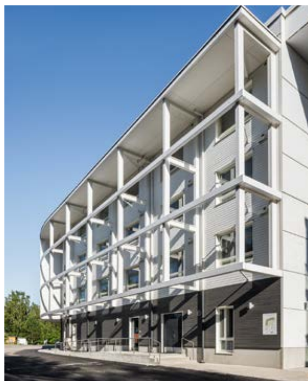
► Nursing and care home – Helsinki (FI)
