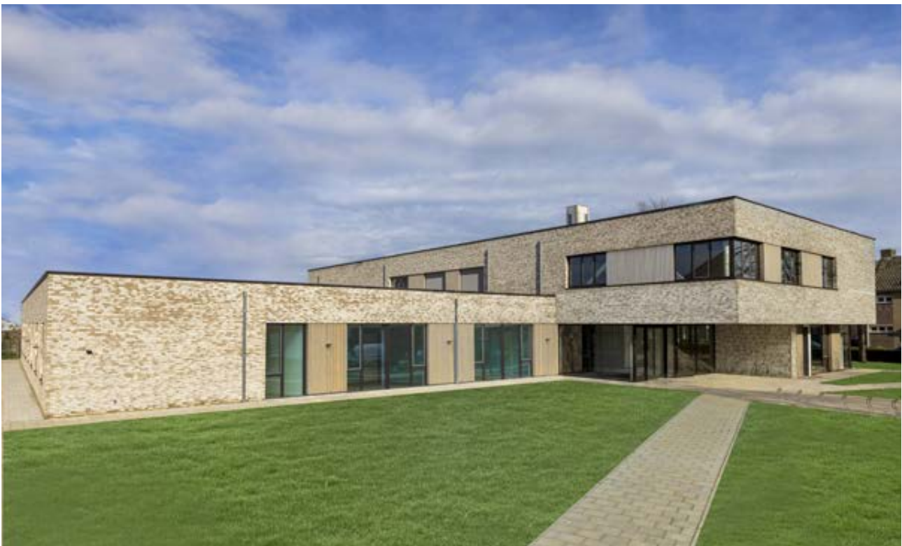
► Medical office building - Sittard (NL)
