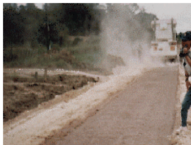
Mechanical Spreading
