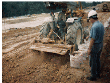
Mixing by Rotorvator
