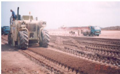
a) Manually Spreading and Mechanically Mixing
