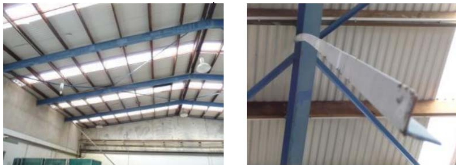
Figure C6.7: Roof bracing that failed during the February 22, 2011 Christchurch earthquake (M. Bruneau)
