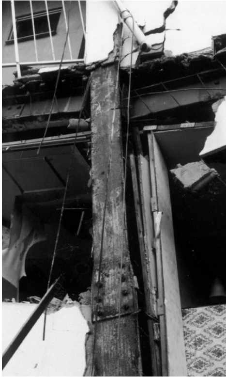
Figure C6A.3: Failed beam to column weak axis welded connection from the 1995 Kobe earthquake
