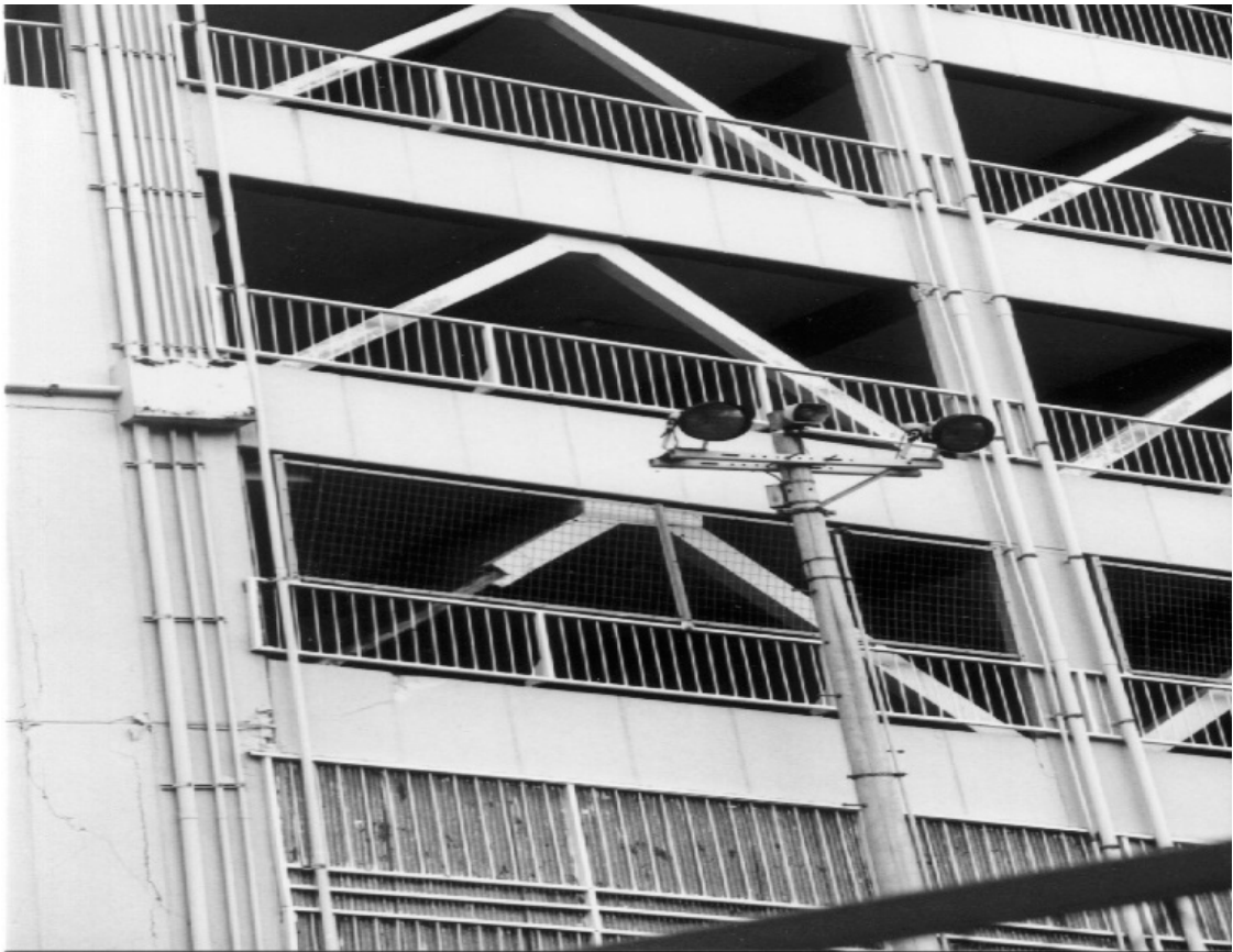
Figure C6A.5: V-braced CBF showing damage but no collapse from the 1995 Kobe earthquake
