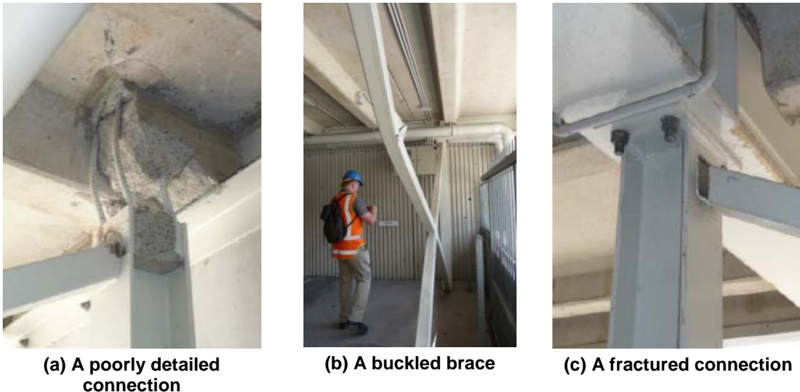
Figure C6.5: Damaged CBFs in a single-storey car park building during the February 22, 2011 Christchurch earthquake (M. Bruneau)
