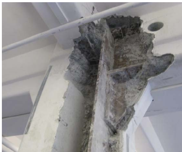
Figure C6.1: A typical riveted beam-column connection
