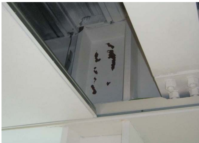
Figure C6.3: Panel zone of an MRF showing minor inelastic action (G.C. Clifton)
