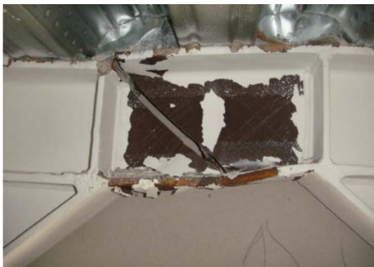
(a) A fractured active link in a 12 storey building
