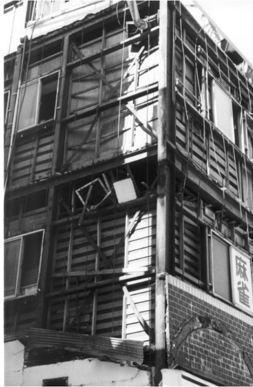
Figure C6A.4: Braced frame with light tension bracing showing damage but no collapse from the 1995 Kobe earthquake
