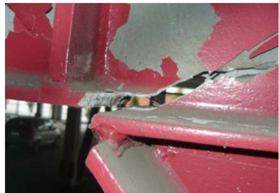
(b) A fractured active link in a low-rise parking building
