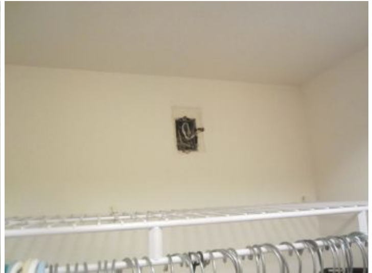
Open junction box in master closet.
