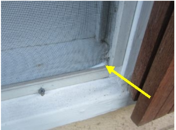
Damaged window screen
