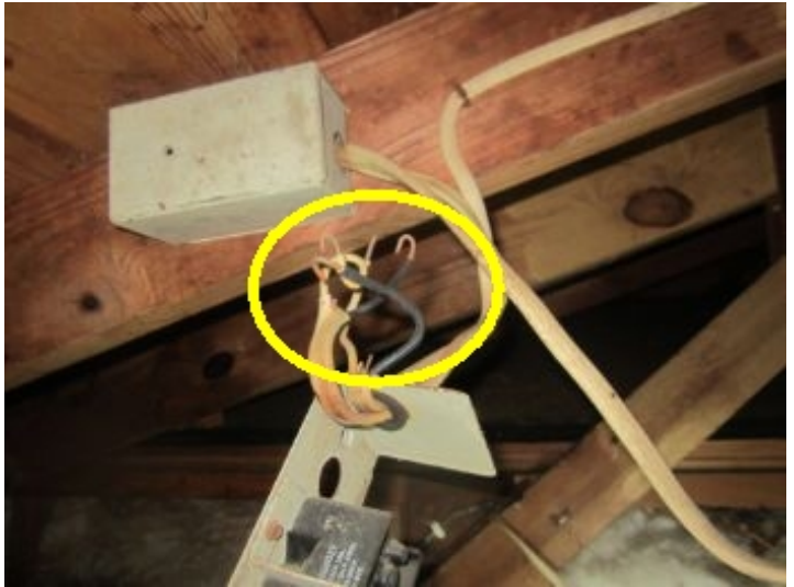
Exposed open-ended conductors in attic
