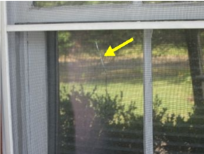
Crack in window
