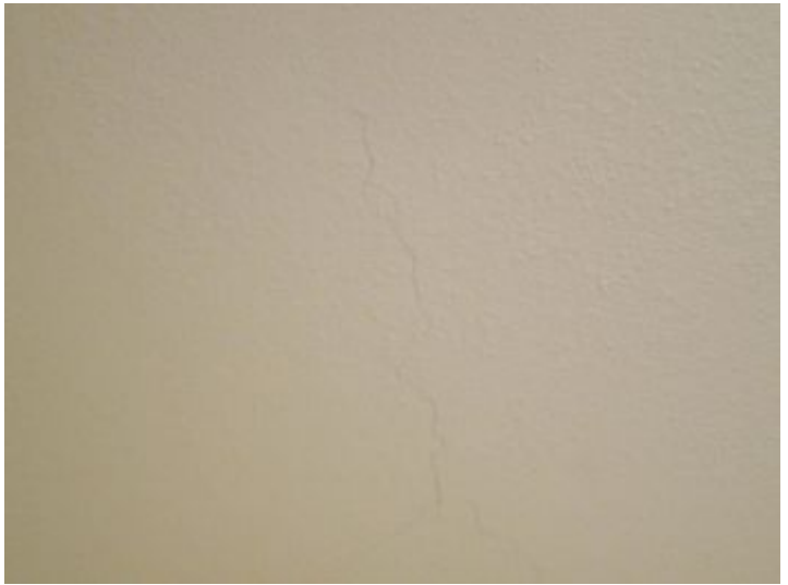
Small crack in 2nd bedroom ceiling
