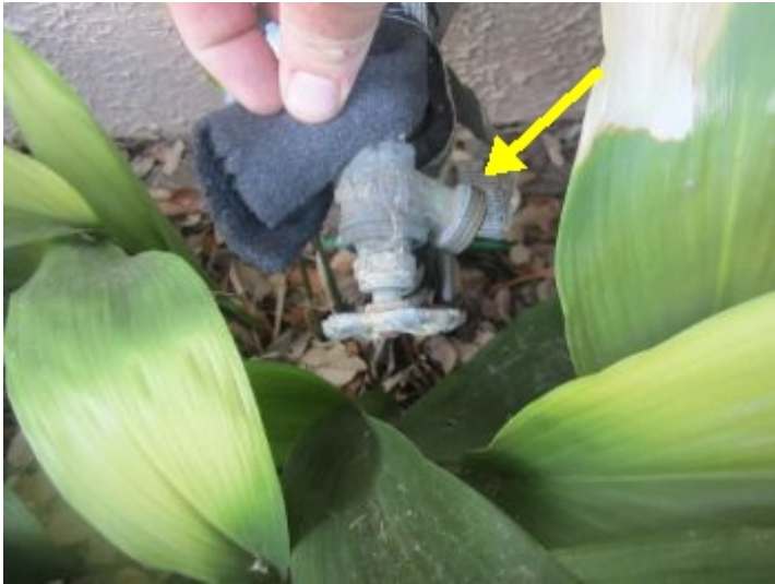
Missing anti-siphon device
