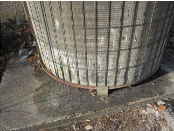
Damaged condenser fins
