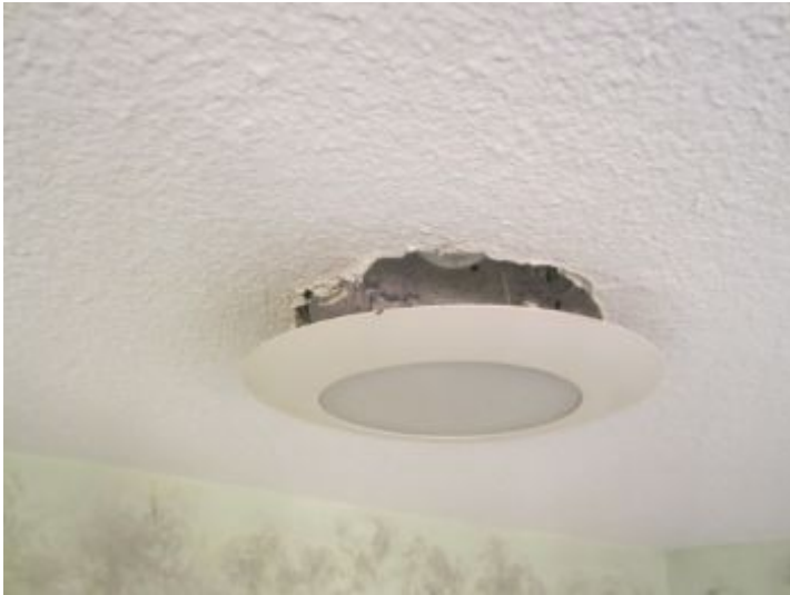
Loose lighting fixture in hallway bath
