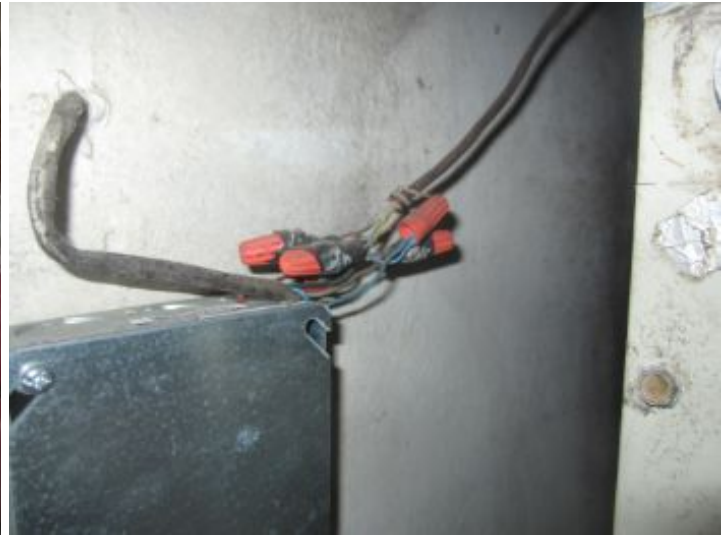
Wire splices not located in J-box
