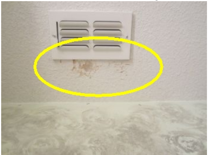
Water spot in hallway bath ceiling
