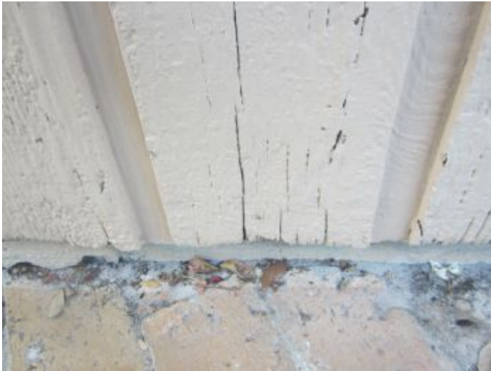
Wood rot on wood paneling of detached garage
