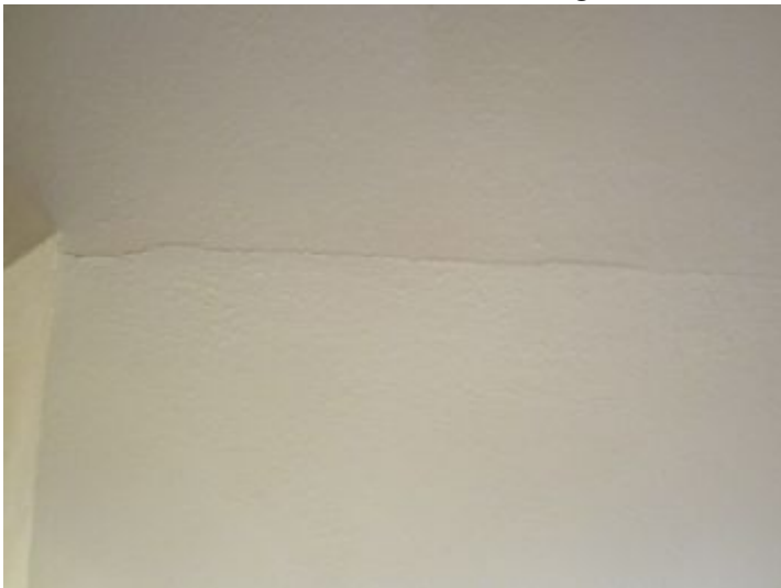
Small crack in hallway ceiling
