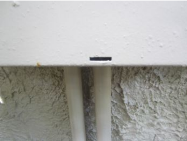
Broken door latch at service panel
