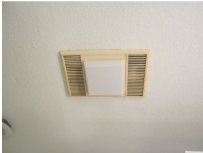
Non-fuctioning light at vent in hallway bath
