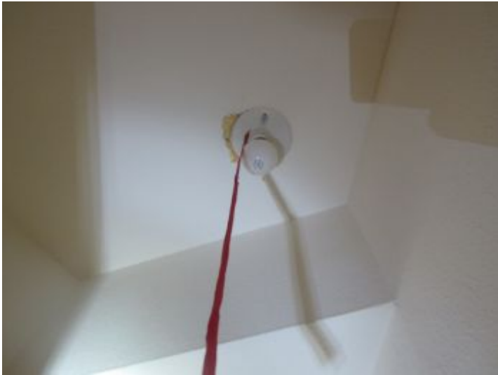
Unprotected light fixture
