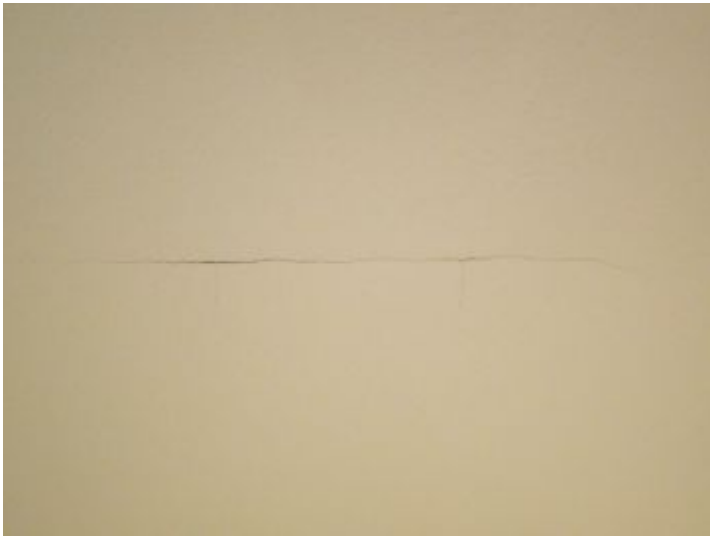
Small crack in master bed ceiling
