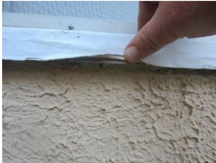
Paint peeling on window sills
