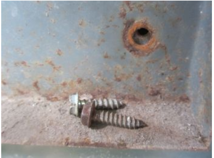
Improper screw type in panel
