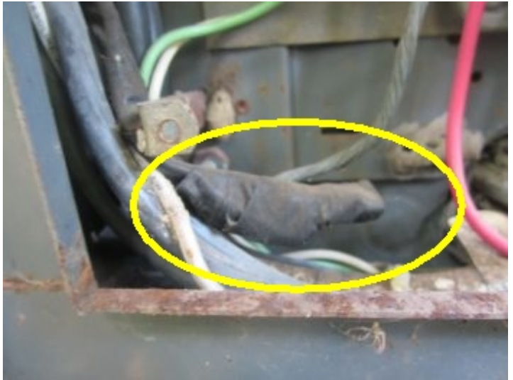
Taped off wiring inside service panel
