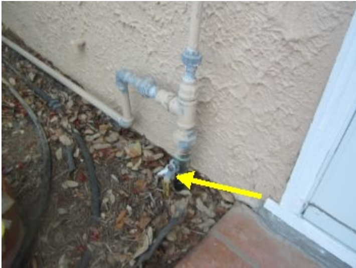
Location of main water supply shut off
