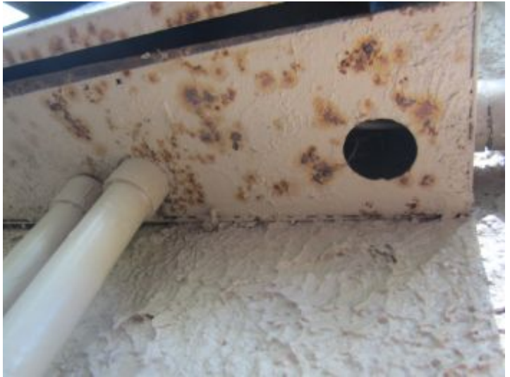
Open knockout at service panel
