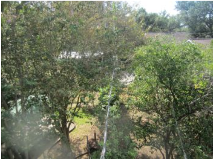
Tree branches in contact with service entrance conductors
