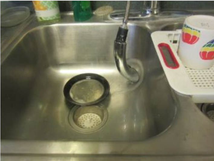
Sprayer is not self-retracting
