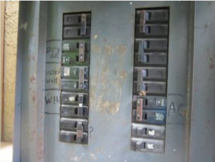
Breakers not completely and properly labeled
