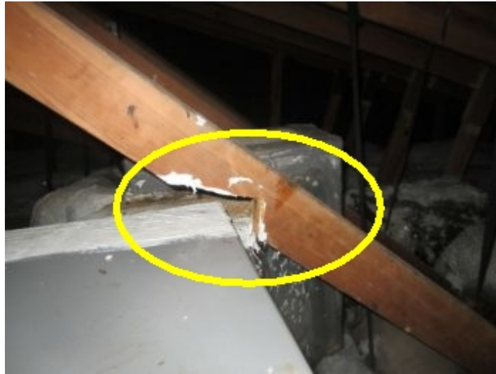
Excessively notched truss in attic at AC unit
