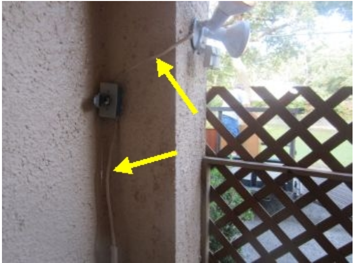
Romex wiring not located inside conduit
