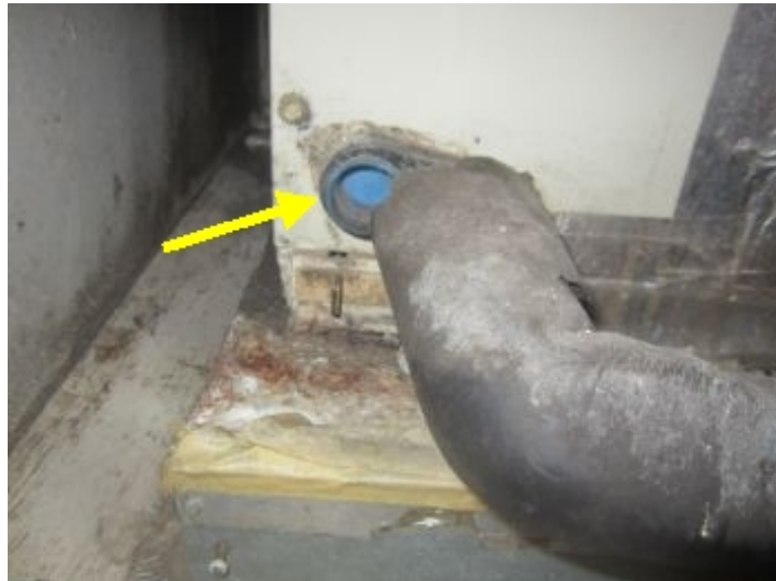
No secondary condensate drain
