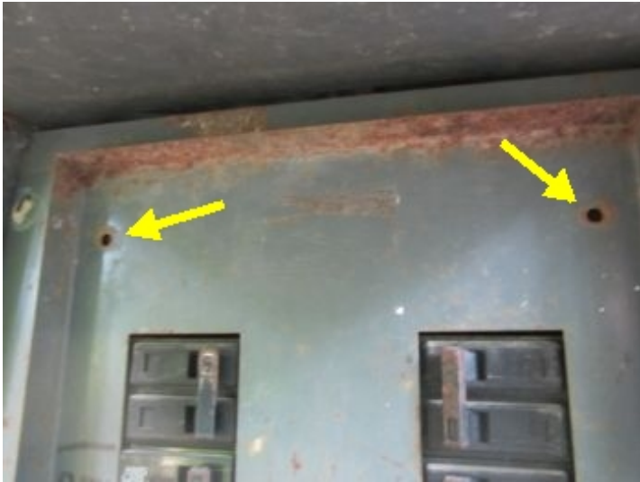
Missing screws in dead front cover
