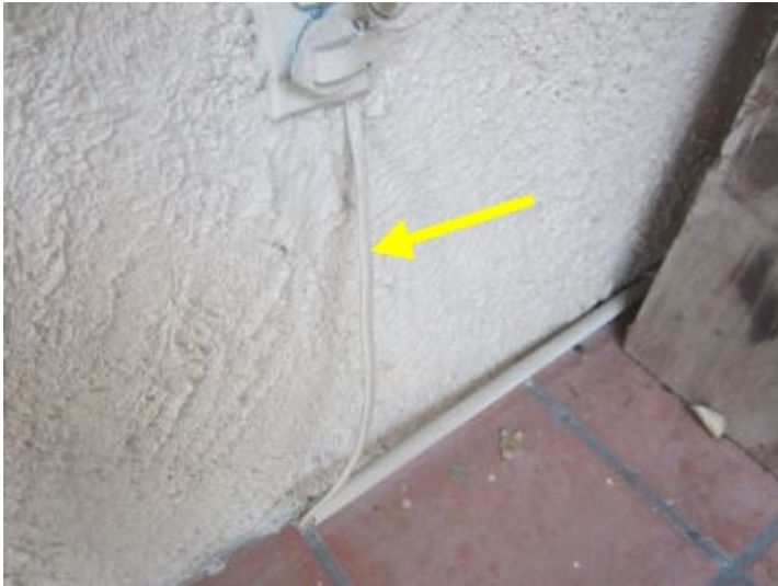
Romex wiring not located inside conduit
