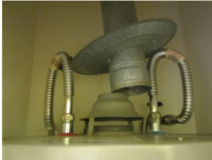
Disconnected B-Vent
