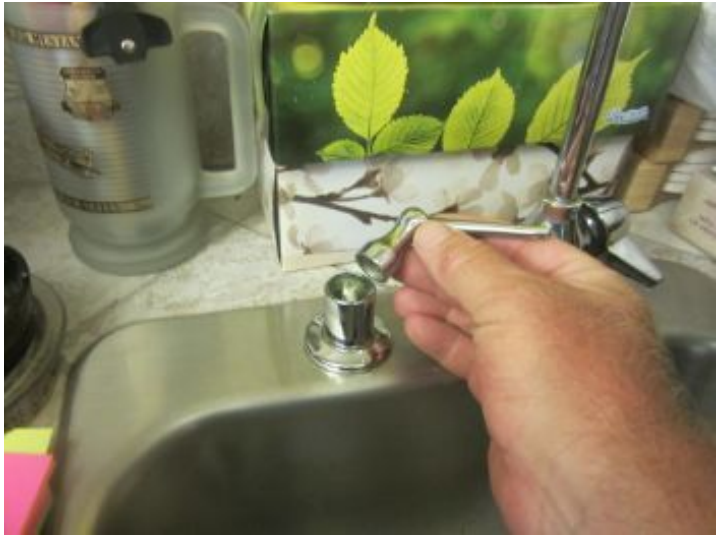
Broken soap dispenser on wet bar sink
