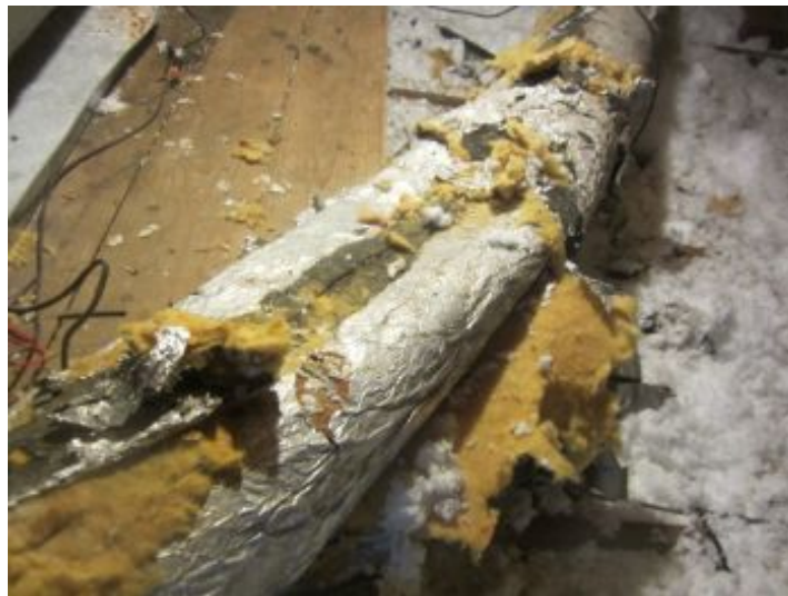
Damaged vent insulation
