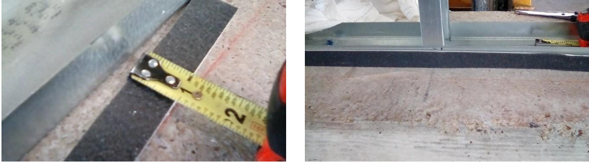
Figure 2: On the left the STS-FRG 75 is shown to be 1 inch wide. On the right the STS-FRG 75 is shown adhered to the floor runner/bottom track.
